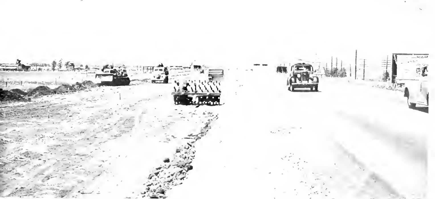
Views of realigned U. S. 40 between Davis and Dixon in Yolo County. Upper—Looking toward Yolo Causeway and Sacramento from point near State Nursery, showing resurfacing material windrowed in center of old highway. Center—Looking toward Davis; State Nursery on left. Bottom—Fill and widening operations for divided highway at point directly south of Yolo Causeway
